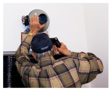
Ben Matter, assisted by apprentices Joel Matter and Rich Mathes, spent a May week installing ventilation (a fan) in addition to using the server room air conditioner to create a system to keep the equipment around 77 degrees.
