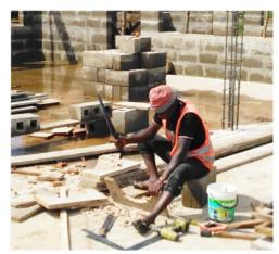
the crew has started to construct the columns to support the roof of the cafeteria and classroom corridor. It's impressive to see how they manage to construct the forms for cylindrical columns with only a straight hand saw and a large knife.
